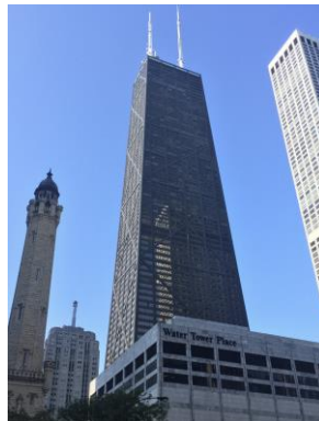
Building Heating and Cooling Wire
