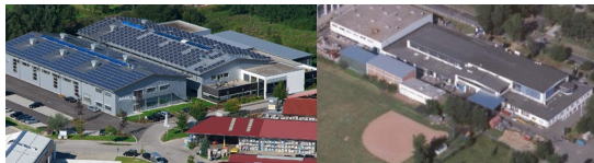
AMAG components, Germany
