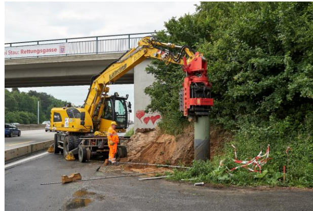
Bringing in the steel tubes as foundation
