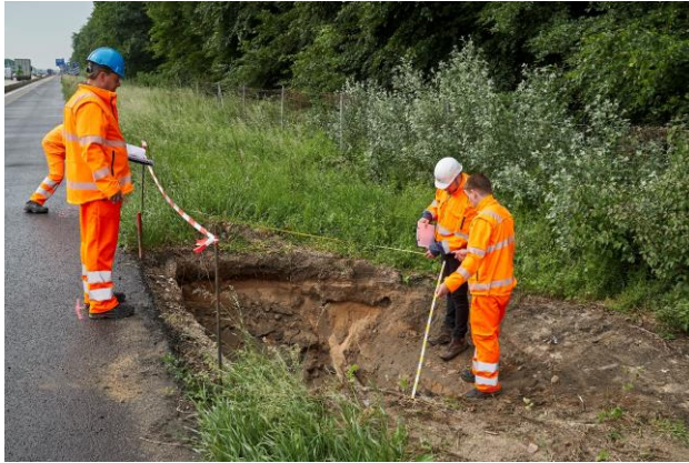
Search shafts checking on underground wires and pipes
