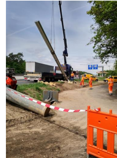
Setting up the poles
