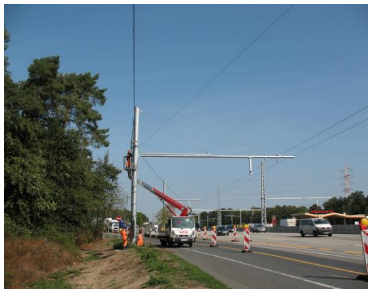
Installation of the cantilevers
