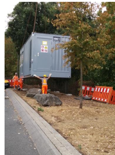
Connecting the substations
