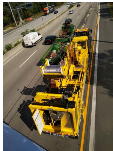
Pulling the wires
